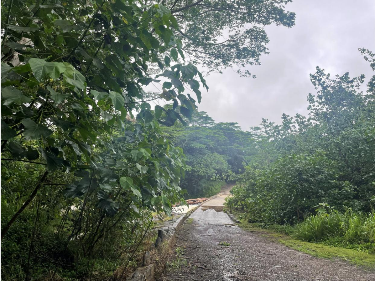
Camera #2 – Christian Crossing Bridge, Kalepa Ag Lands (22°02'13.62" N 159°22'45.10" W) 257 ft. Elevation
